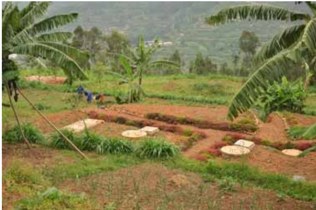
Figure 4.5: Biogas Digesters at Rulindo High School
